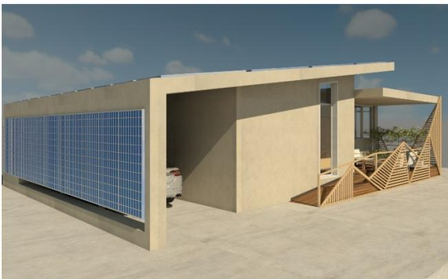
Fig. 10. Side PV panels used as shades to the Garage
